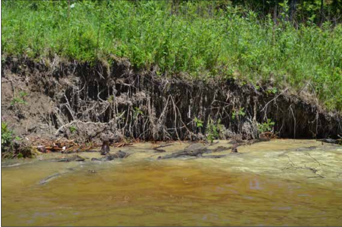
Figure 16. Headwall erosion at site 21SL898, June 2014.
