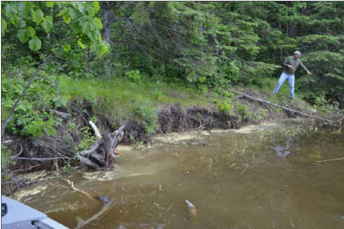
Figure 19. Terrace headwall at site 21SL38, June 2014.
