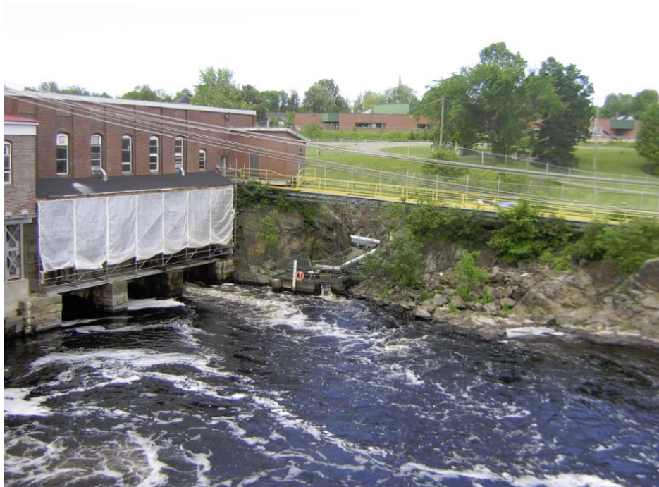
Milltown Dam (6-15-2016) View of Powerhouse with Enclosure on Tailrace Wall and Fishway Below Dam.
