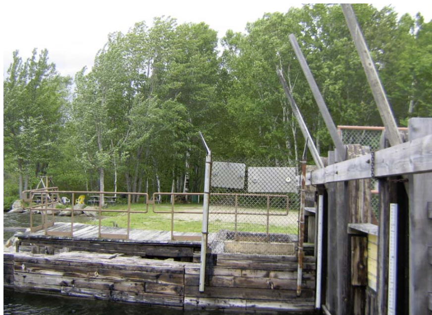
Forest City Dam (6-15-2016) View of Wooden Sluice Gates at Dam (Upstream) and Adjacent Fishway.
