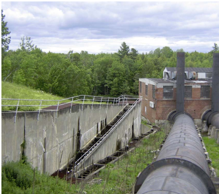
Grand Falls Dam (6-15-2016) View of Denil Fishway Alongside Powerhouse.
