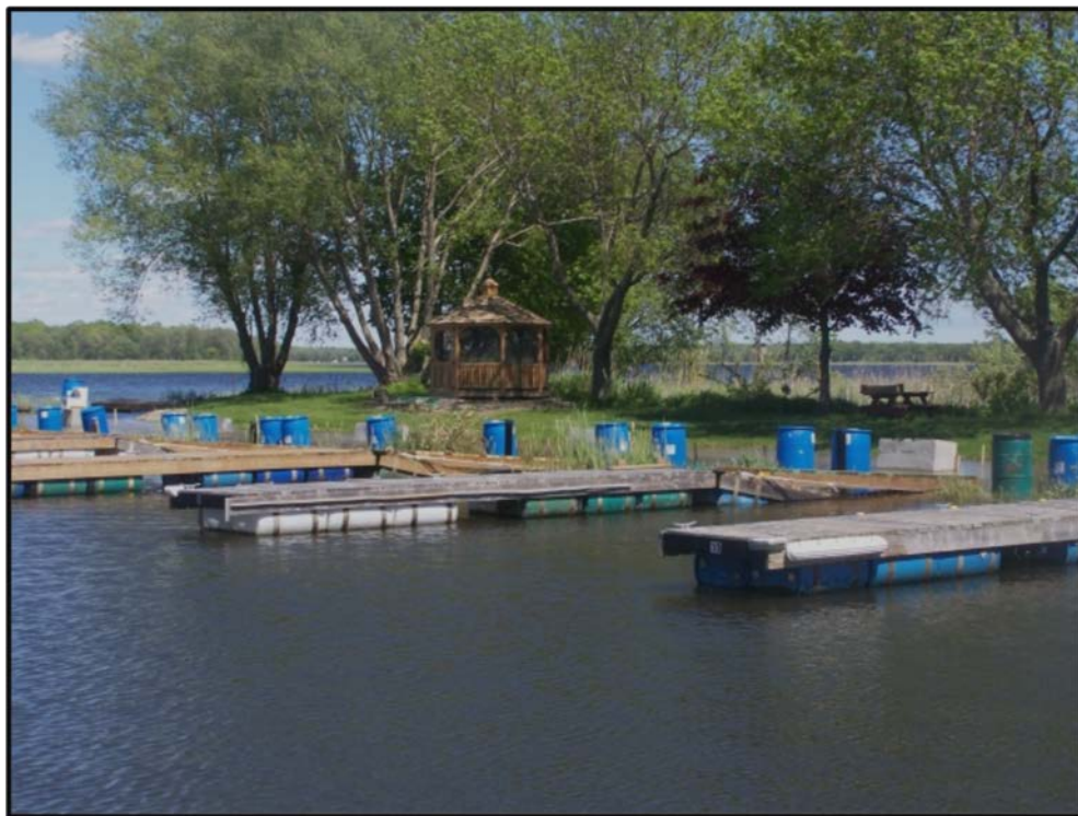
Figure 8-31: New floating docks installed at the Presqu'île Yacht Club in Brighton, ON. Action taken to adapt to extreme water levels such as those experienced in May and June 2017. Photo credit: http://presquileyc.com/high-water-project-update/
