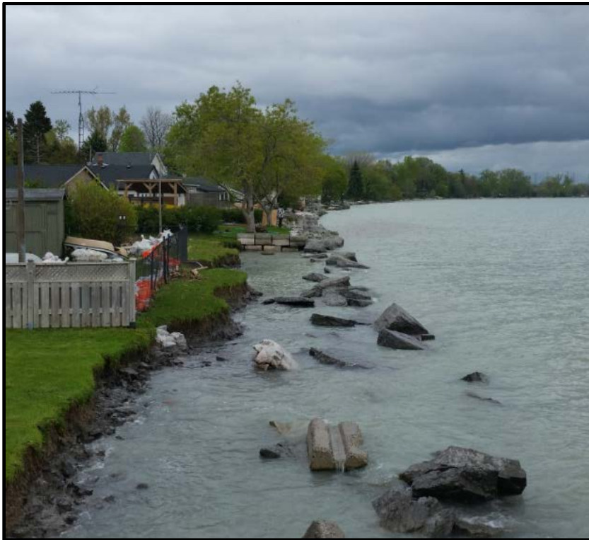
Figure 6-50: Shoreline erosion behind failed shoreline protection in Municipality of Clarington, May 26, 2017. Photo credit: Municipality of Clarington Fire and Emergency Services.
