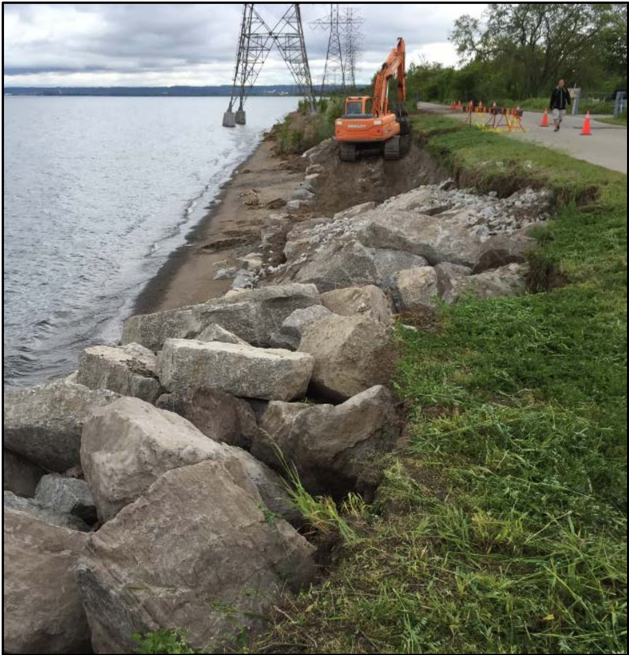
Figure 6-80: Emergency shore protection installation to protect a portion of Hamilton's waterfront trail from erosion on June 1, 2017. Photo credit: ECCC.
