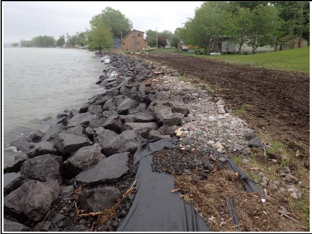
Figure 3-4: Additional rip rap placed to protect sanitary sewer line in Sodus Point observed on 26 May 2018 Photo credit: USACE Buffalo, 2017.
