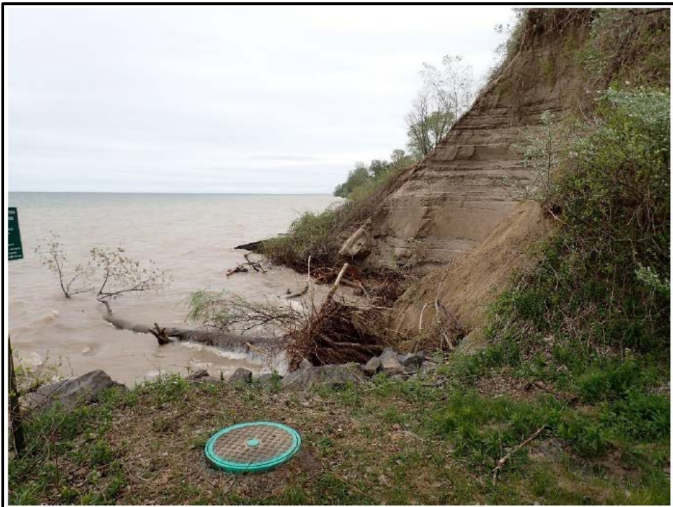
Figure 3-3: Bluff erosion approximately 10 ft. from WWTP outfall, in Sodus Point, NY, 19 May, 2017. Photo credit: USACE Buffalo, 2017.
