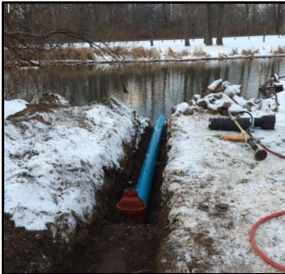
Figure 3-9: Installation of pipes and shut-off valve in Greece, NY as a flood response (Source: WHAM, Rochester, February 5, 2018 - http://13wham.com/news/local/greece-adds-new-pipes-valves-in-high-risk-flood-locations )
