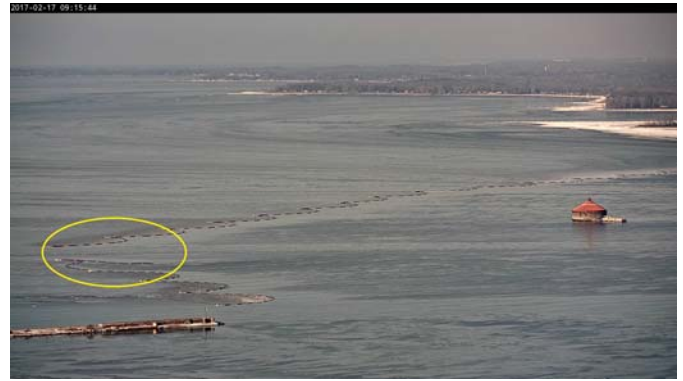
Figure 5: Span E is circled in yellow, shown open and trailing. Image courtesy of NYPA from the Lake Erie-Niagara River Ice Boom webcam.
