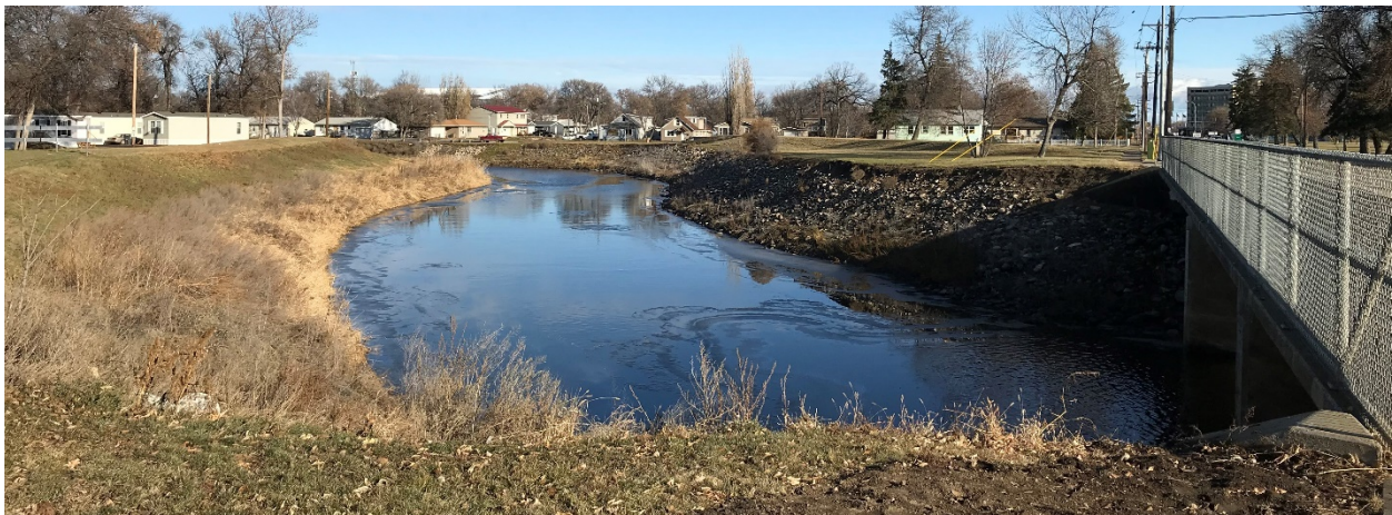
8 th Ave SE Souris River Crossing in Minot, ND. Photo taken by: Darrell Corkal
