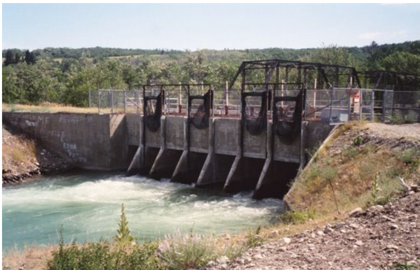
St. Mary Diversion Dam
