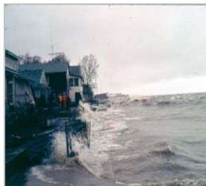
Figure above is of high water levels on Lake Ontario in 1973. Photo provided by Baird & Assoc.
