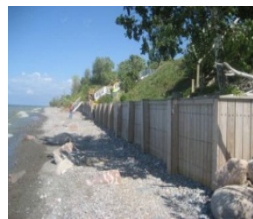
Figure to the left is of a vertical wall shore protection on the south shore of Lake Ontario. Photo provided by AECOM
