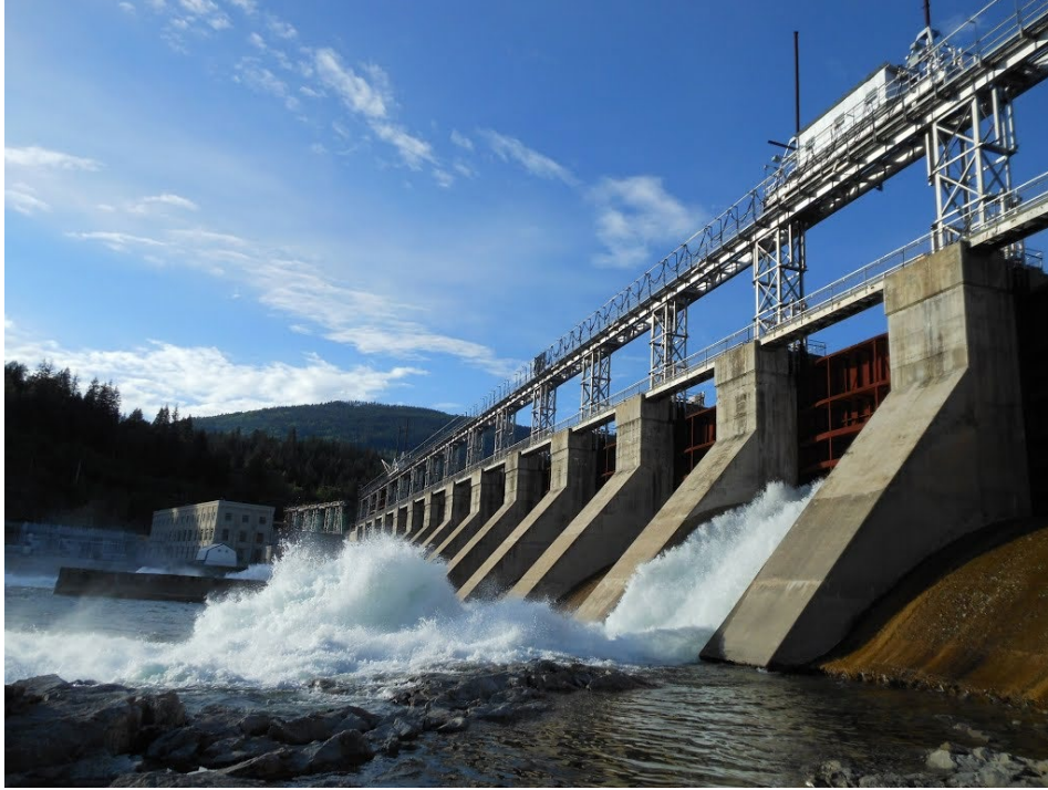
Photograph of Kootenay River free-fall discharge through Corra Linn dam during the Spring high-water period (Photo: Fortis BC)
