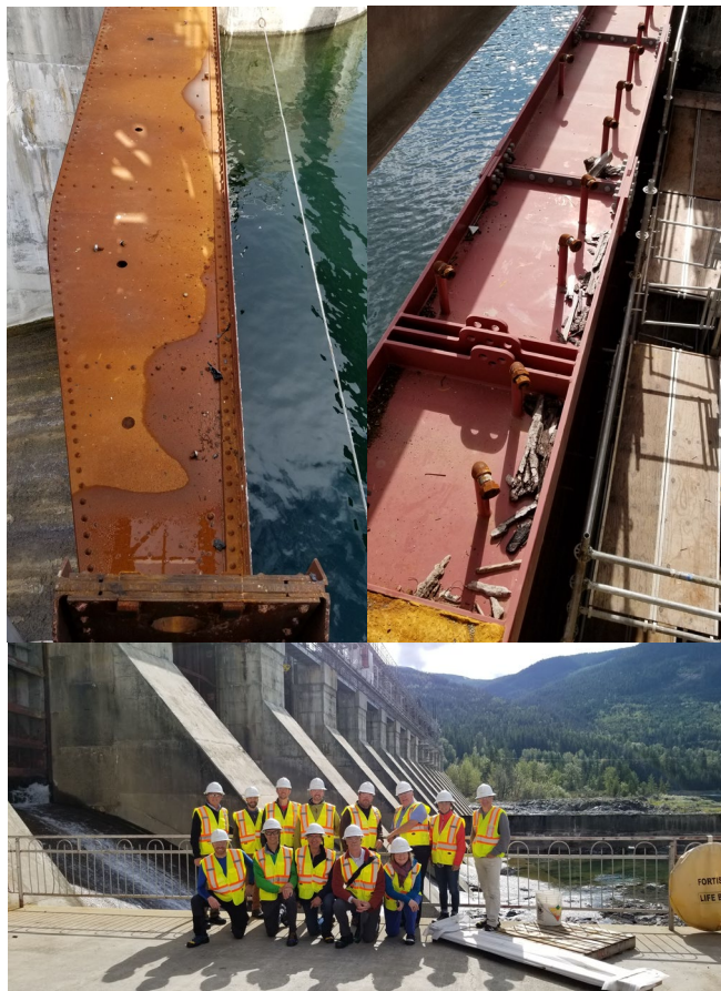
Figure 2 – Clockwise from Top Left: Original Corra Linn Dam spillway gate, Temporary Cofferdam to allow gate replacement, IKLBC and guests group photo. September 19, 2019.
