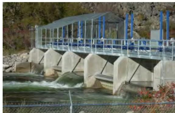
**Figure 2.13:** New overshoot gates at McIntyre Dam to enable fish passage.
