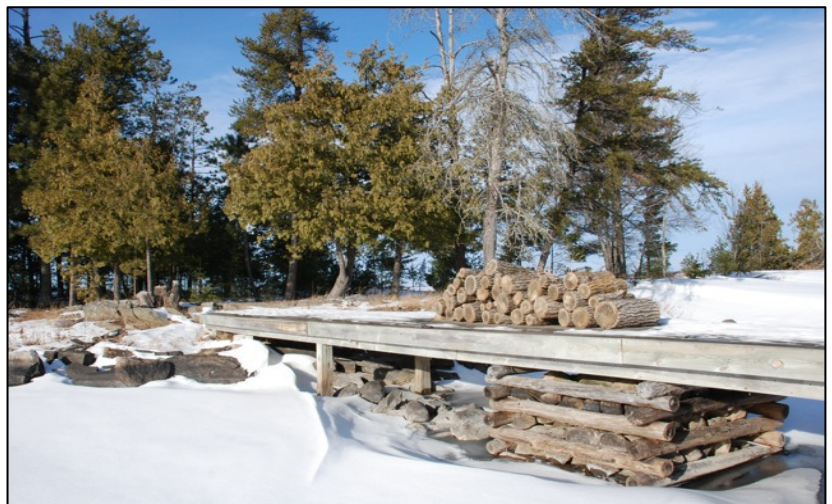
Low Rainy Lake levels leave this dock crib exposed on Minitaki Island in early winter. Photo: Lee Grim
