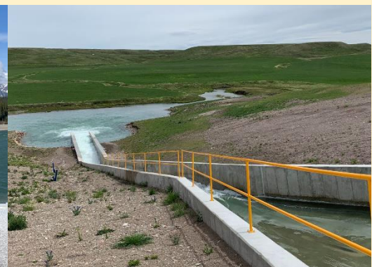
Drop Structure No.5 on the St. Mary Canal (Credit: ECCC Staff)
