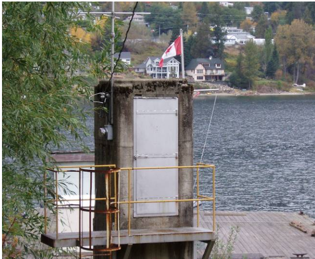
The Kootenay Lake water level recorder gauge house at Nelson, BC.
