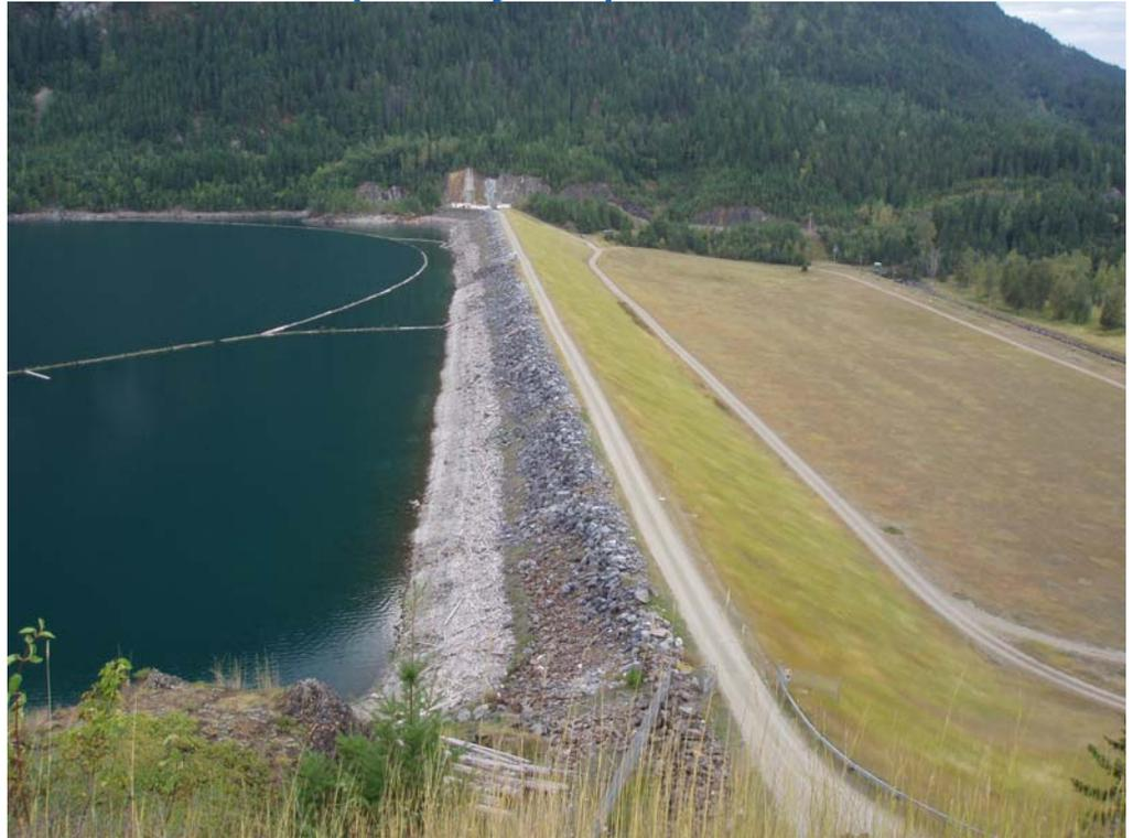
Duncan Dam (BCHydro) was constructed in 1967 as the first of three Canadian dams in British Columbia required under the Columbia River Treaty, creating the Duncan Lake reservoir along the Duncan River, about 10 km upstream of the north end of Kootenay Lake (BC). This Dam does not generate electricity but serves a storage purpose to assist in the optimization of downstream hydroelectric facilities via regulation of flow to Kootenay Lake.
