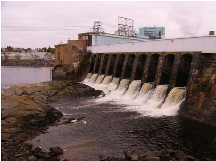
**Figure 3-8 - Gate flow under closed conditions (J. Bruxer, 2009)**
