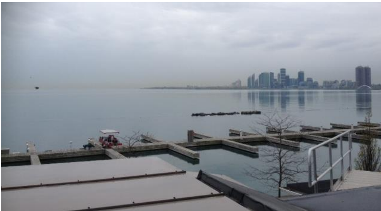
Image 7: Breakwall completely submerged, providing no protection of the docks and grounds from waves. (Photo Credit: The Boulevard Club).
