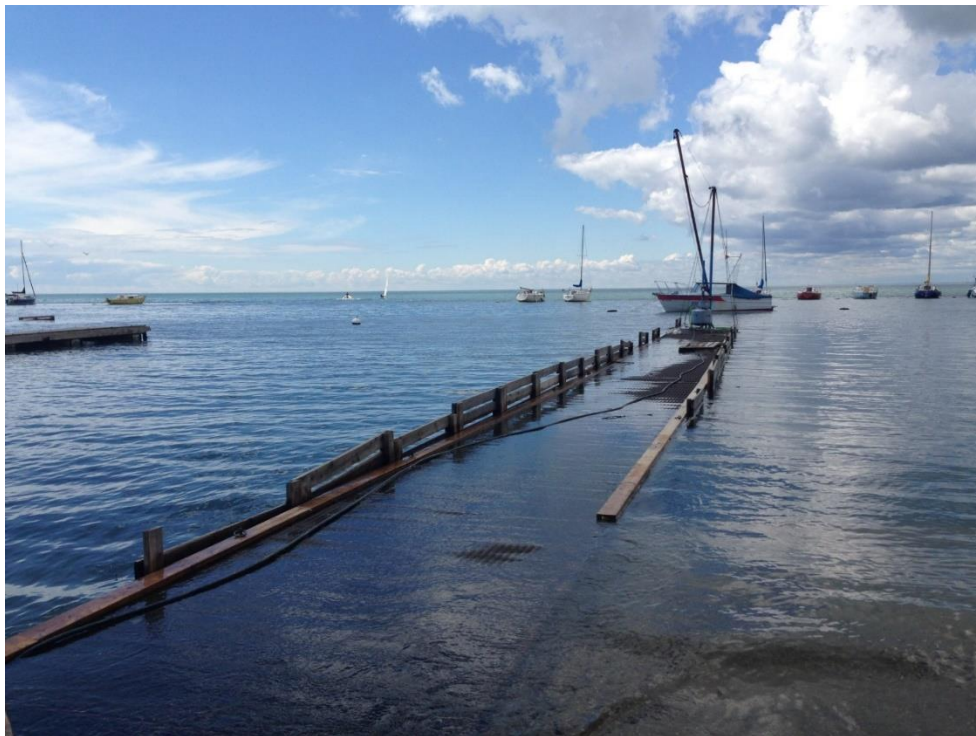
Image 3: Flooding of a fixed dock (Photo Credit: Anonymous, Toronto Sailing & Crane Club)
